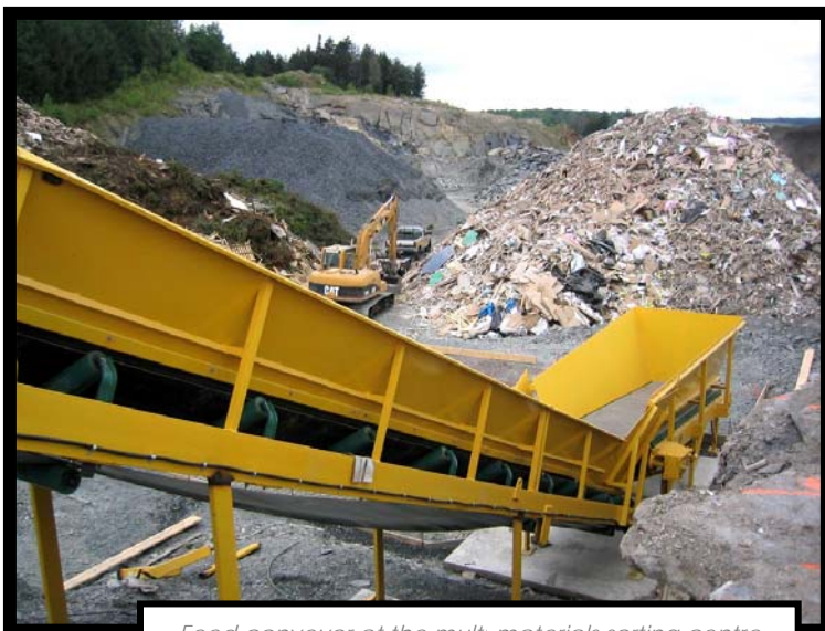
Feed conveyor at the multi-materials sorting centre
